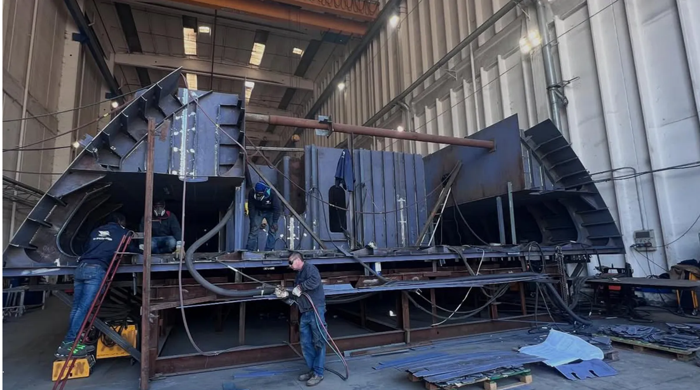
FB291 entered construction in 2025 - Credit: Joe Foggia
